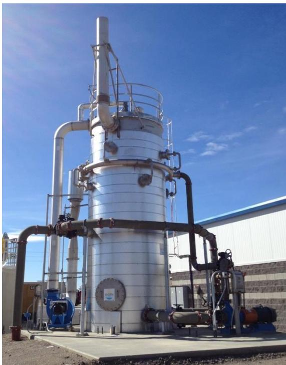
gases. The wastewater is circulated from the bottom of the tank to the head space by a centrifugal pump and a set of non-clog spraying nozzles.
